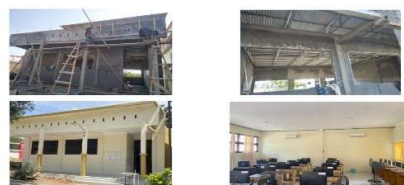
Figure 7. Construction of the Computer Laboratory
