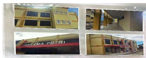
Figure 4. Boys' and Girls' Dormitory Buildings
