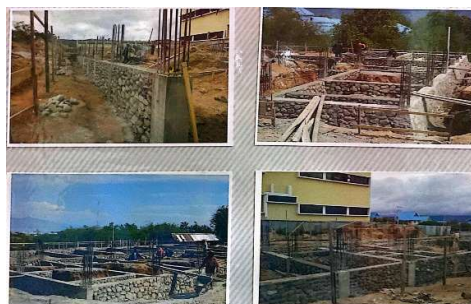
Figure 2. Construction of the Main School Building
